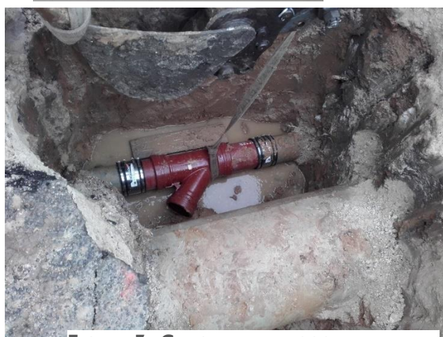
FIGURE 7 : CULOTTE DE RACCORDEMENT
